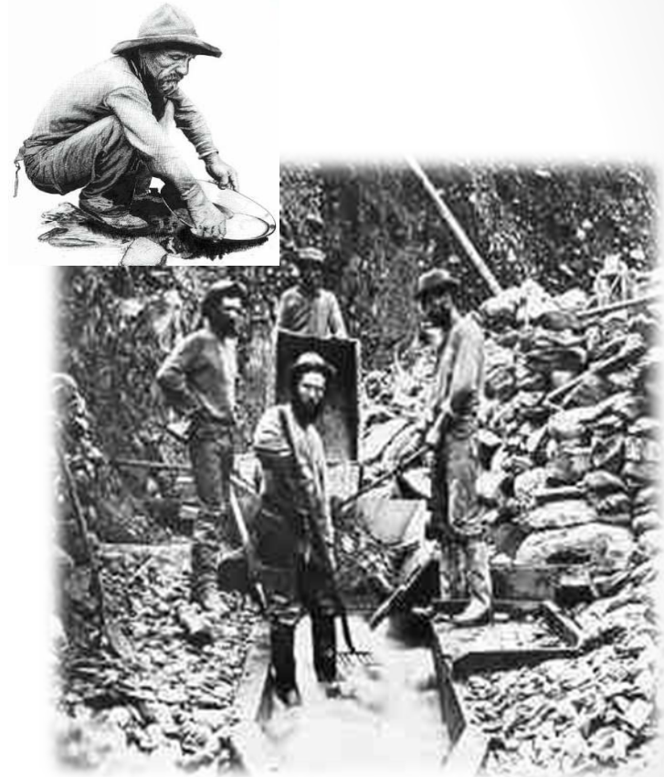
Miners, ground sluicing, Grouse Creek, 1867 or 1868. ( British Columbia Archives and Records Service, HP765 ).
