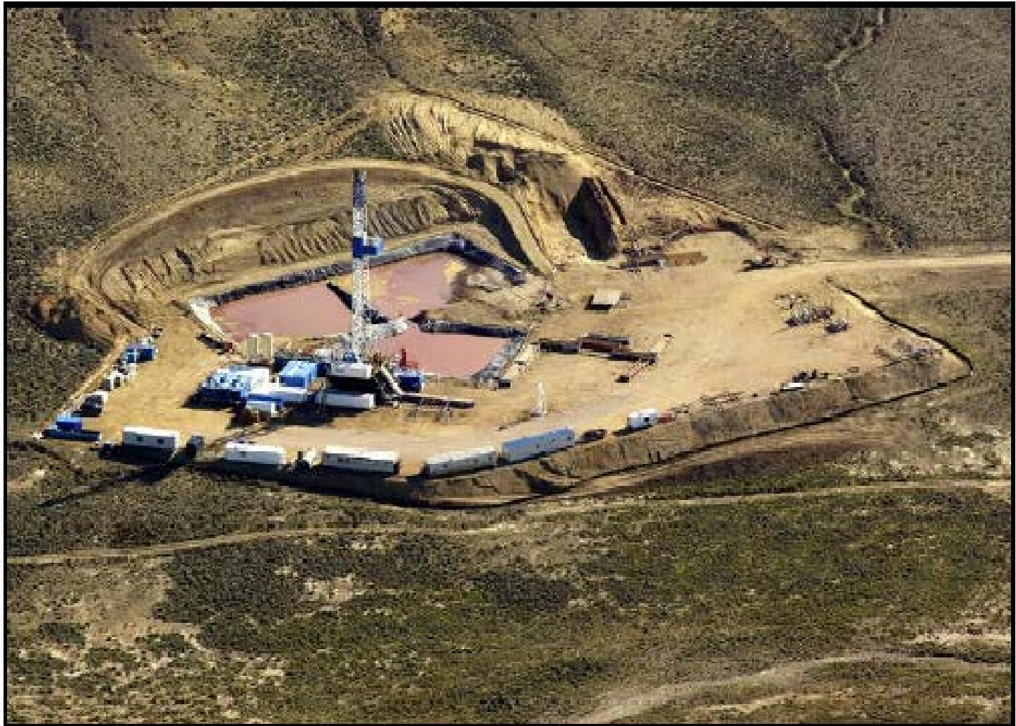
Figure 1. Photograph taken in 2002 of a gas well being drilled on a typical well pad. Note pits containing drilling fluids, equipment trailers, and access road.
